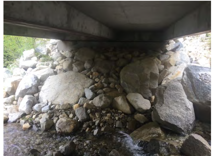
Right Bank Abutment when facing downstream
