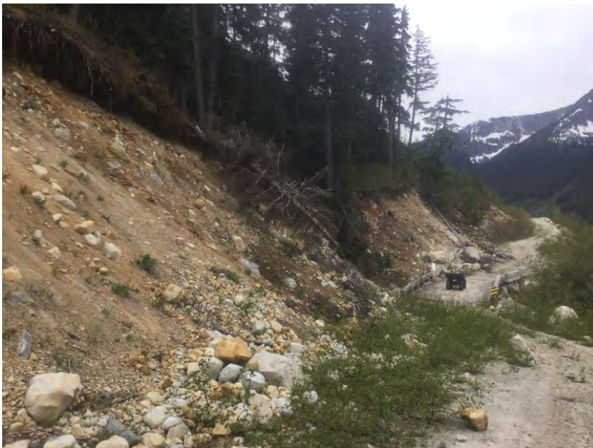
Ravelling cutslope sat both approaches
