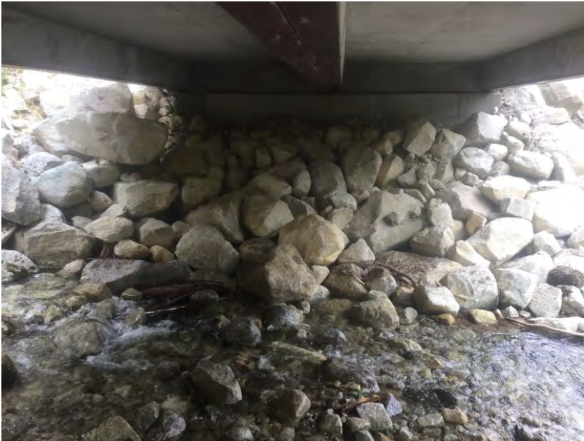
Left Bank Abutment when facing downstream
